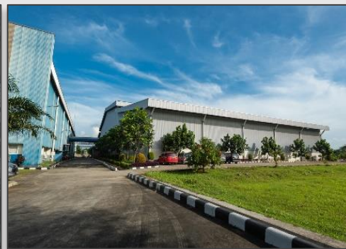
Plant 3 - Logistic center Bekasi, Indonesia
