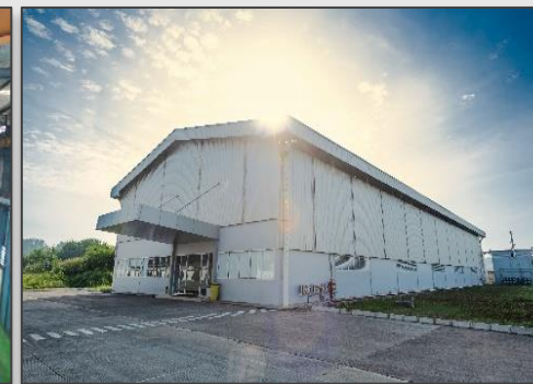
Factory plant 5 Bekasi, Indonesia
