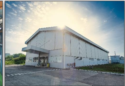
Factory plant 5 Bekasi, Indonesia
