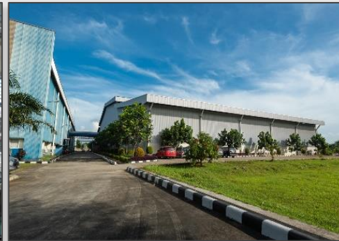
Plant 3 – Logistic center Bekasi, Indonesia
